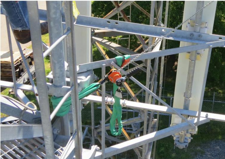
Ensure that all boom components, to include mast pipe and attachment components, are free of damage due to stress, rust, or other potential damage types.
