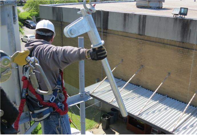
Antenna mast pipe, attachment points to the boom, and boom attachments must be inspected prior to installation of the Lite Gin Pole to ensure all connectins are up to relevant standards.
